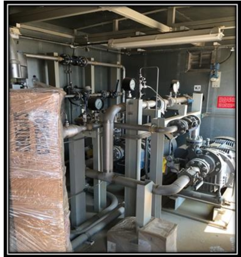
Water Injection Skid
