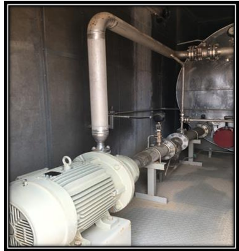
Compressor Wash Enclosure
