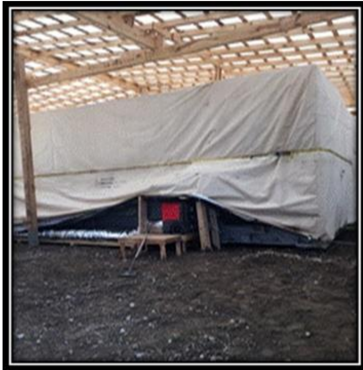
7EA Gas Turbines Under Preservation
